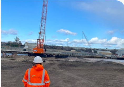
Crawler crane dockside
