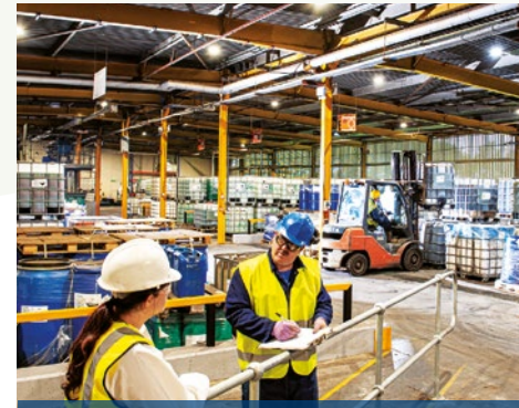
Augean's Berwick-upon-Tweed Hazardous Waste Treatment Facility
